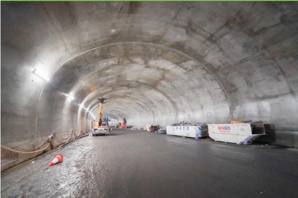
Final lining complete
