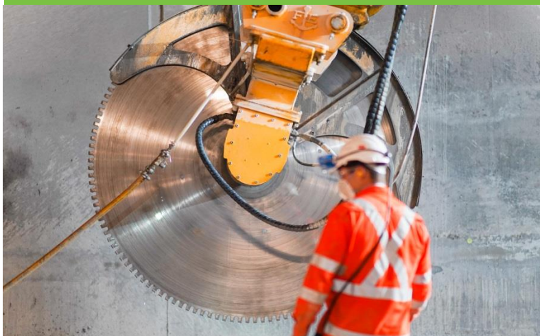
Inspecting the saw cutter used for trenching
